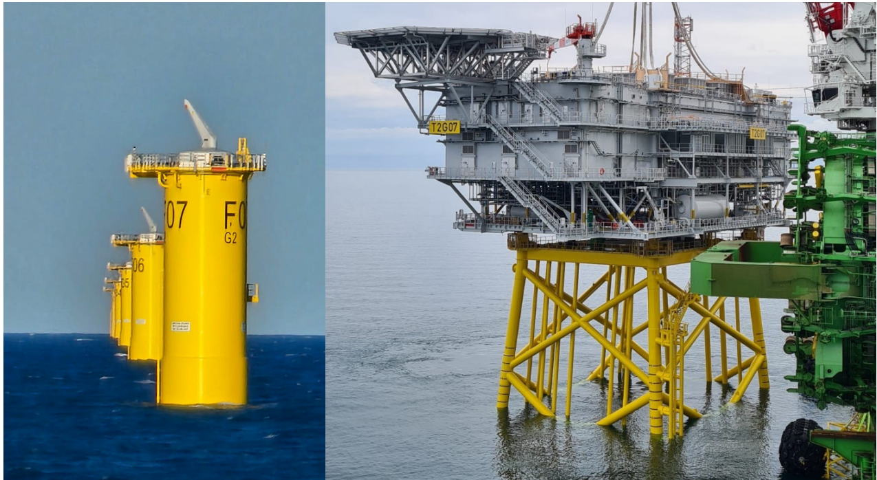
Figure 4: Installed Transition Pieces (TP) along "Row F" spaced 0.9-miles apart and Offshore Substation with Topside.
