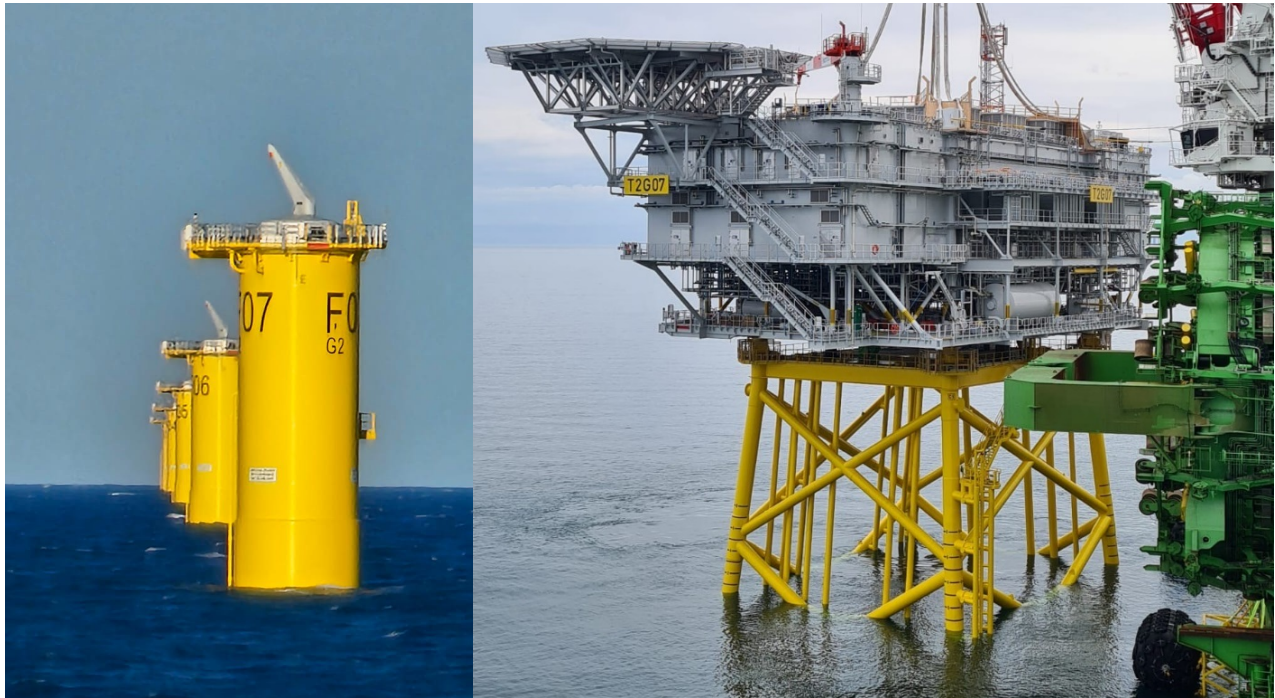
Figure 4: Installed Transition Pieces (TP) and Offshore Substation with Topsides.
