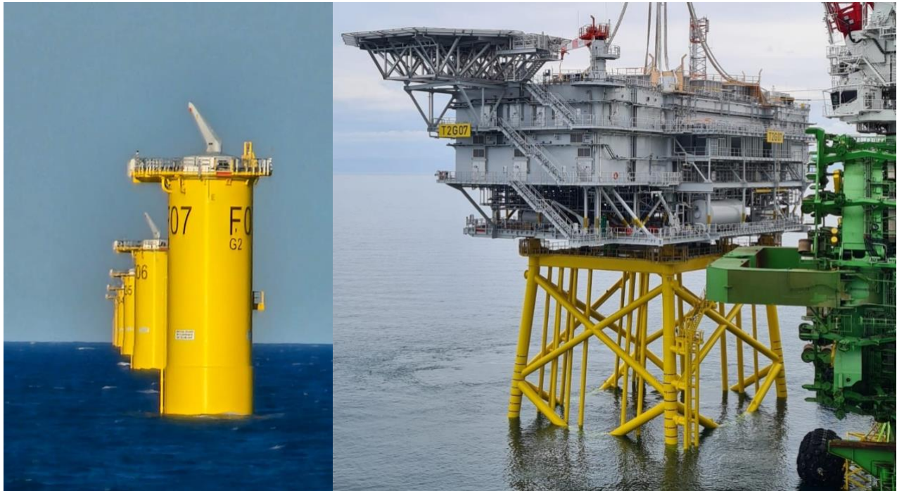
Figure 4: Installed Transition Pieces (TP) and Offshore Substation with Topside.
