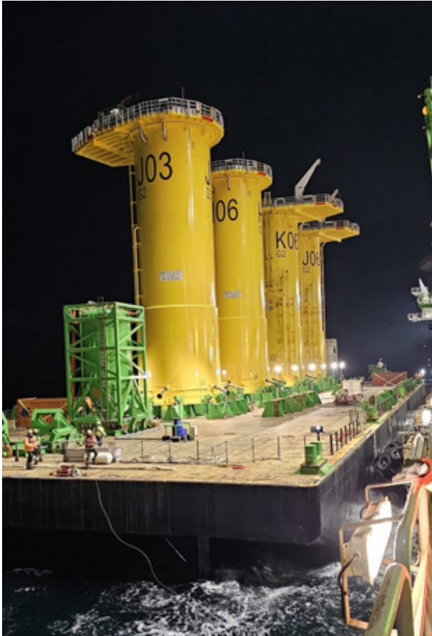
Barge Julie B delivering Transition Pieces to ORION and installed Transition Piece G2K06.
