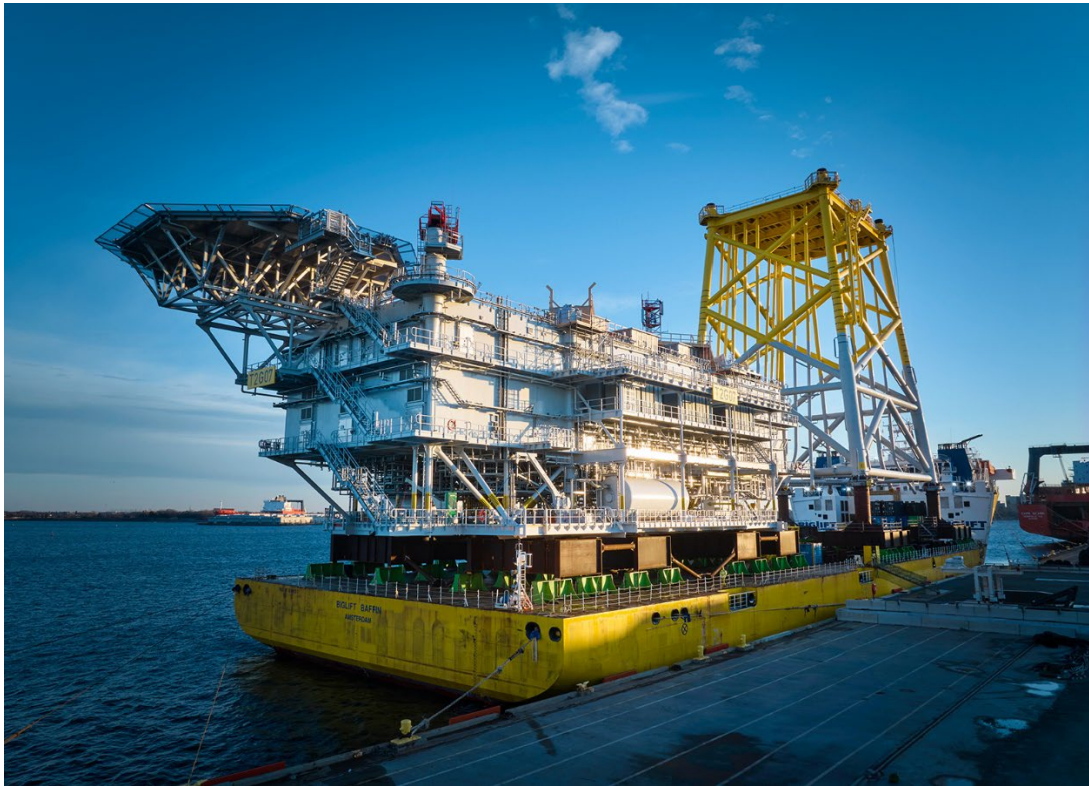
Figure 4: BIGLIFT BAFFIN loaded with the jacket foundation and topside for Offshore Substation (OSS) #2.
