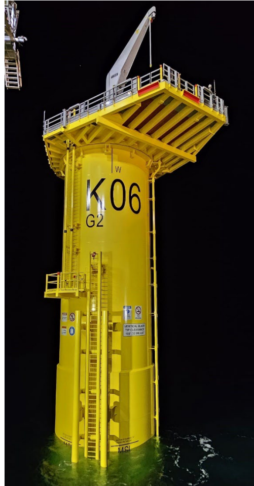
Fig. 6: Transition Piece G2K06 installed
