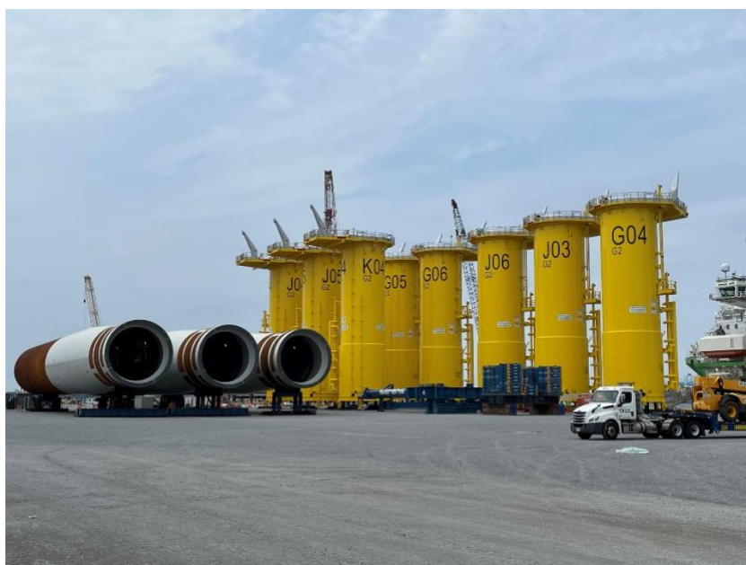
Transition pieces and foundations staged at Portsmouth Marine Terminal
