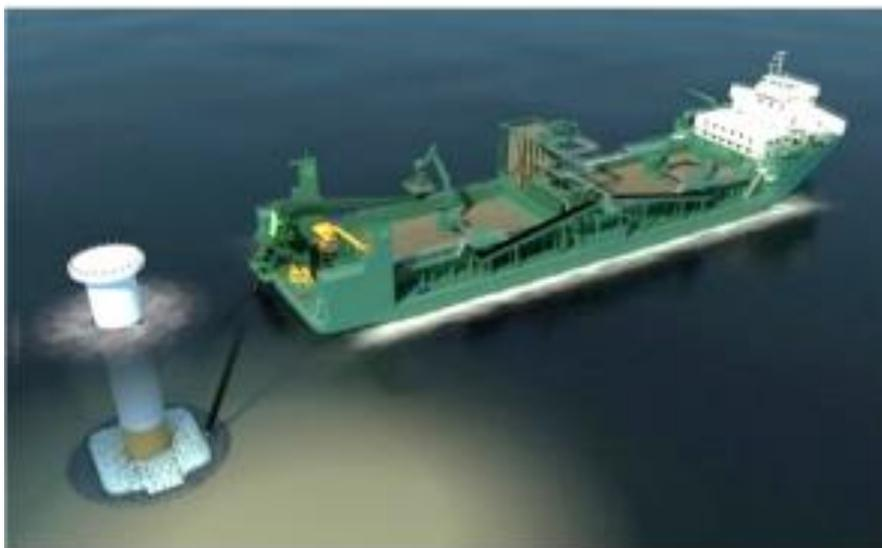
Example of fall pipe vessel installing scour protection
