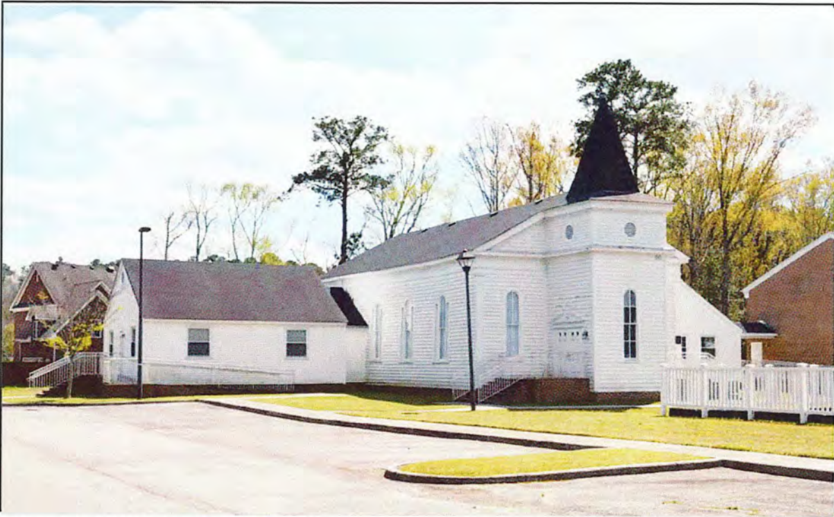
Figure 9: 134-0702, St. John's Baptist Church, north and east elevations, view to the southwest
