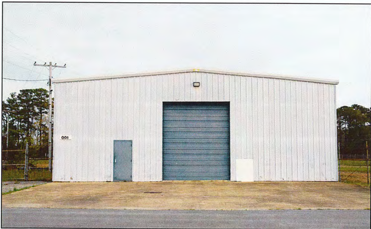
Figure 8: 134-0413-0110, Building 1, south elevation, view to the north.
