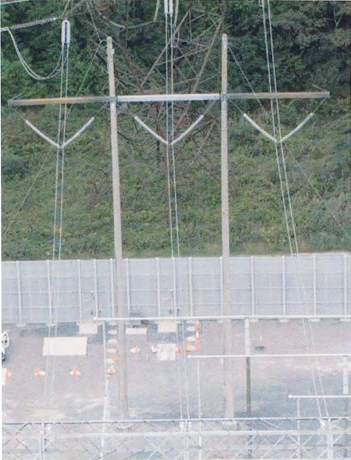
Existing Structure Type: 500 kV Single Circuit H-Frame
