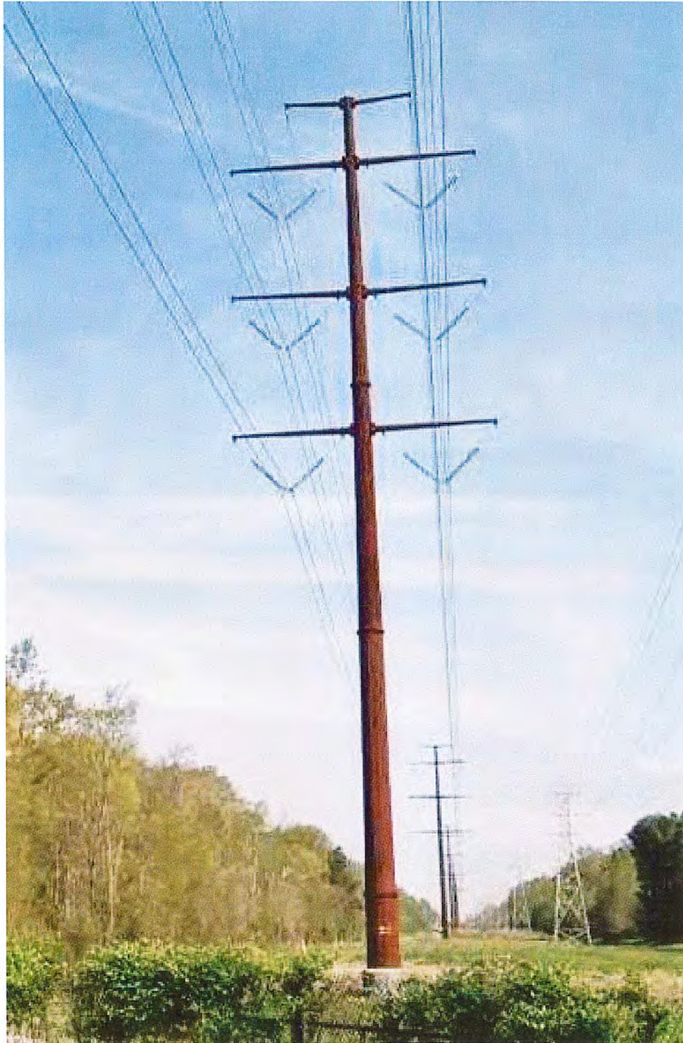
Proposed Structure Type: 230 kV Double Circuit Steel Monopole (Tangent)
