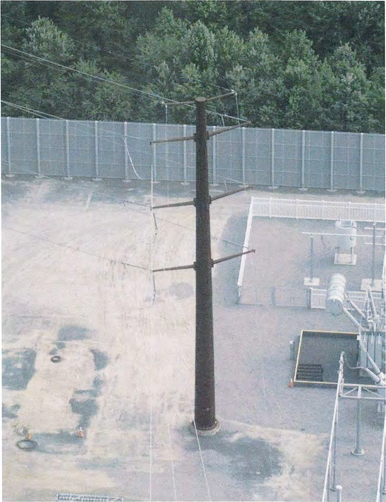
Existing Structure Type: 230 kV Single Circuit Steel Monopole (Double Deadend)
