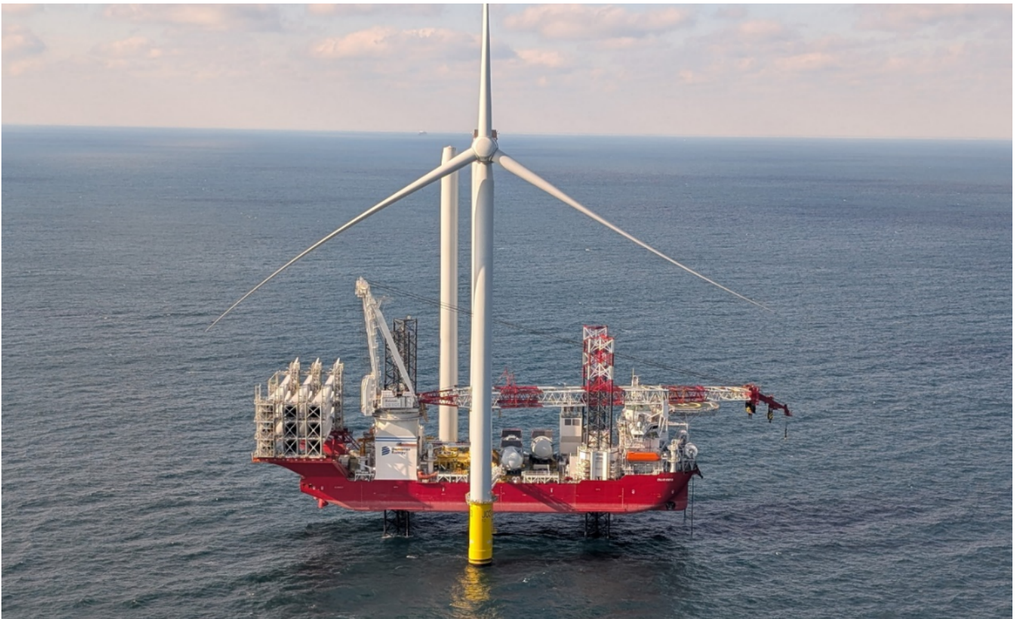
Figure 3: First CVOW Wind Turbine Generator installed by CHARYBDIS
