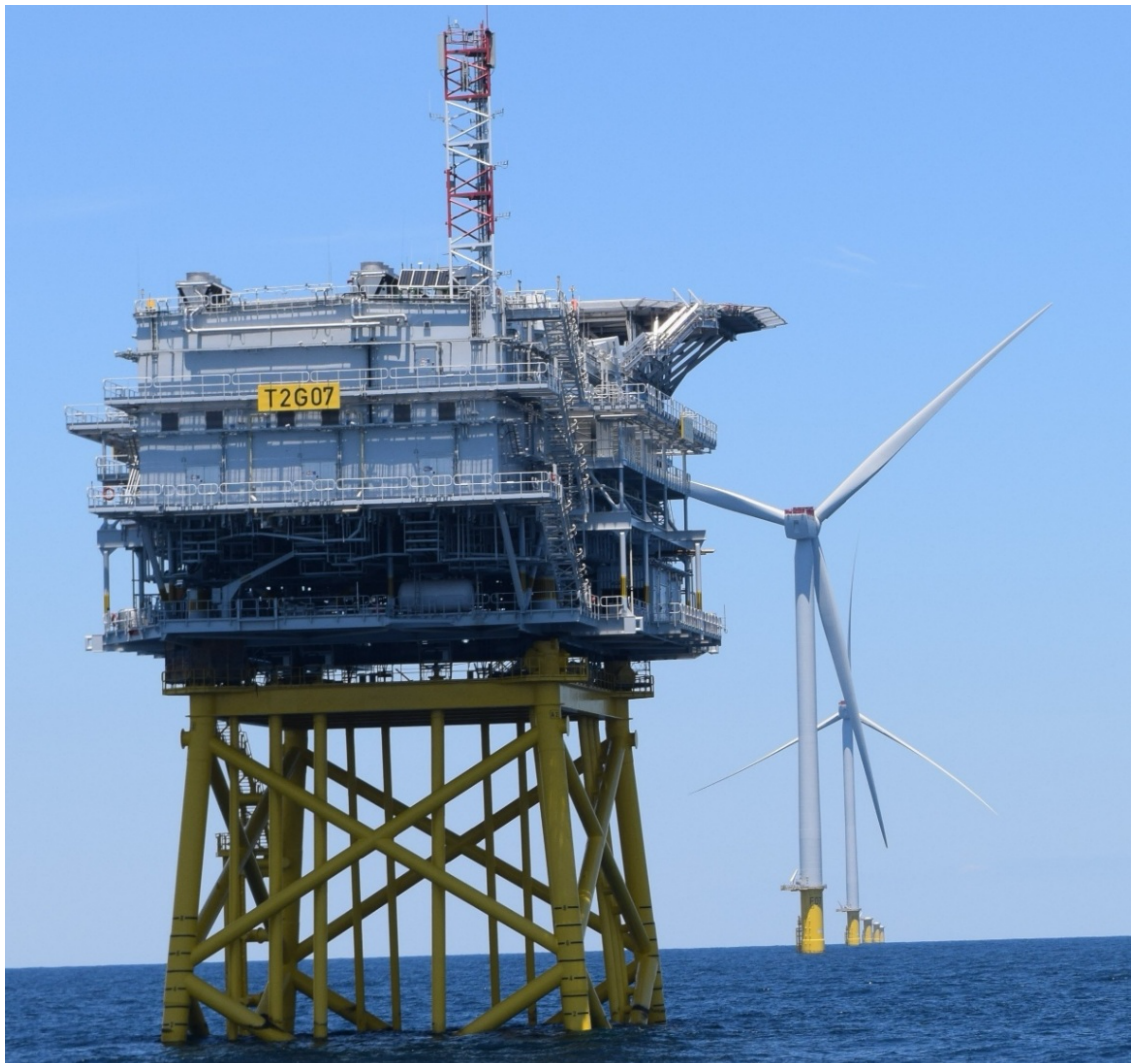
Figure 5: Completed OSS with topside
