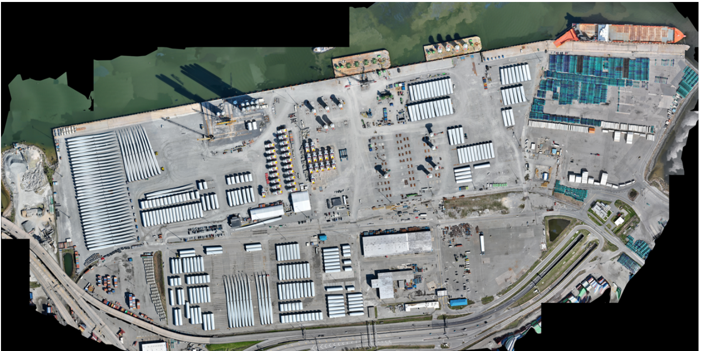
Figure 8: Portsmouth Marine Terminal – Staged WTG Components
