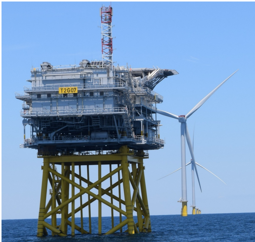
Figure 5: Completed OSS with topside
