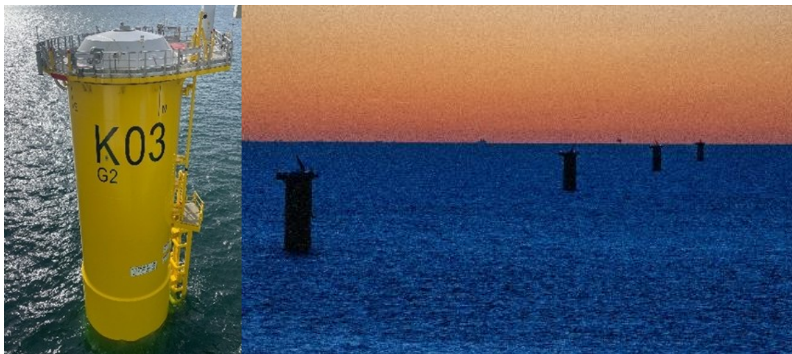
Figure 9: Temporary marine navigation lights on installed TPs
