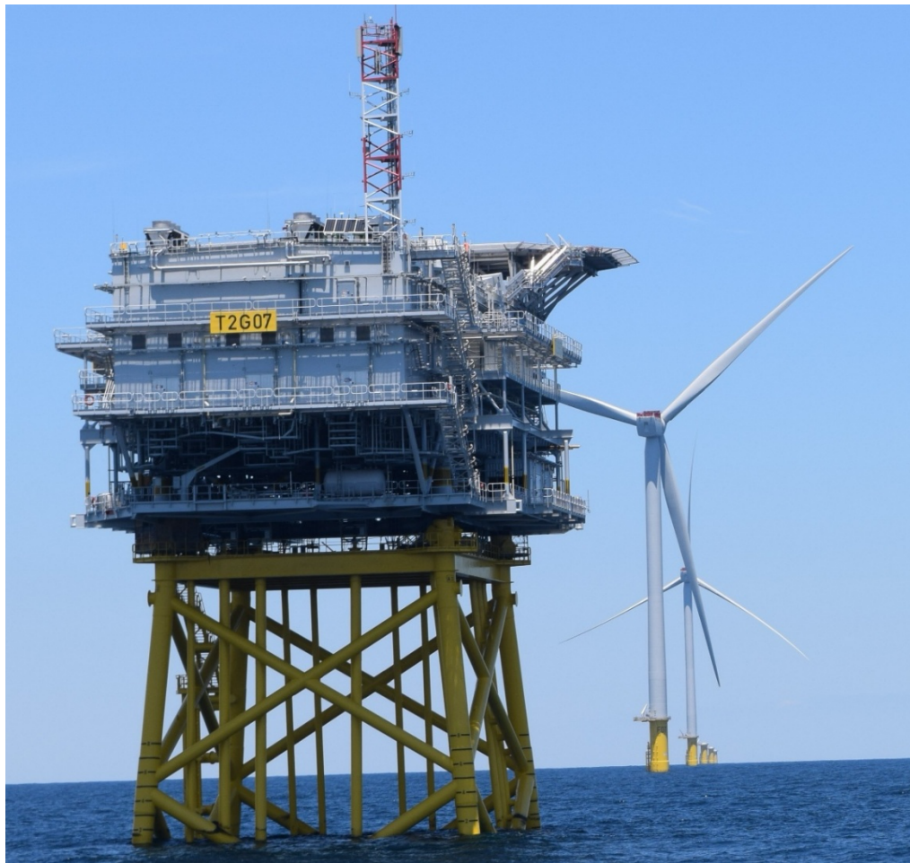
Figure 5: Completed OSS with topside
