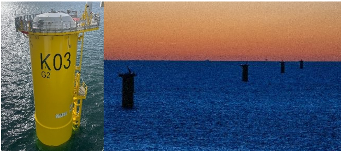
Figure 10: Temporary marine navigation lights on installed TPs
