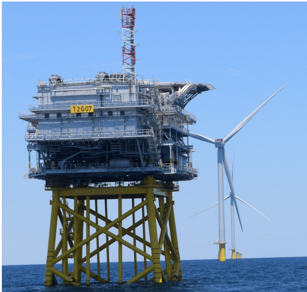
Figure 5: Completed OSS with topside
