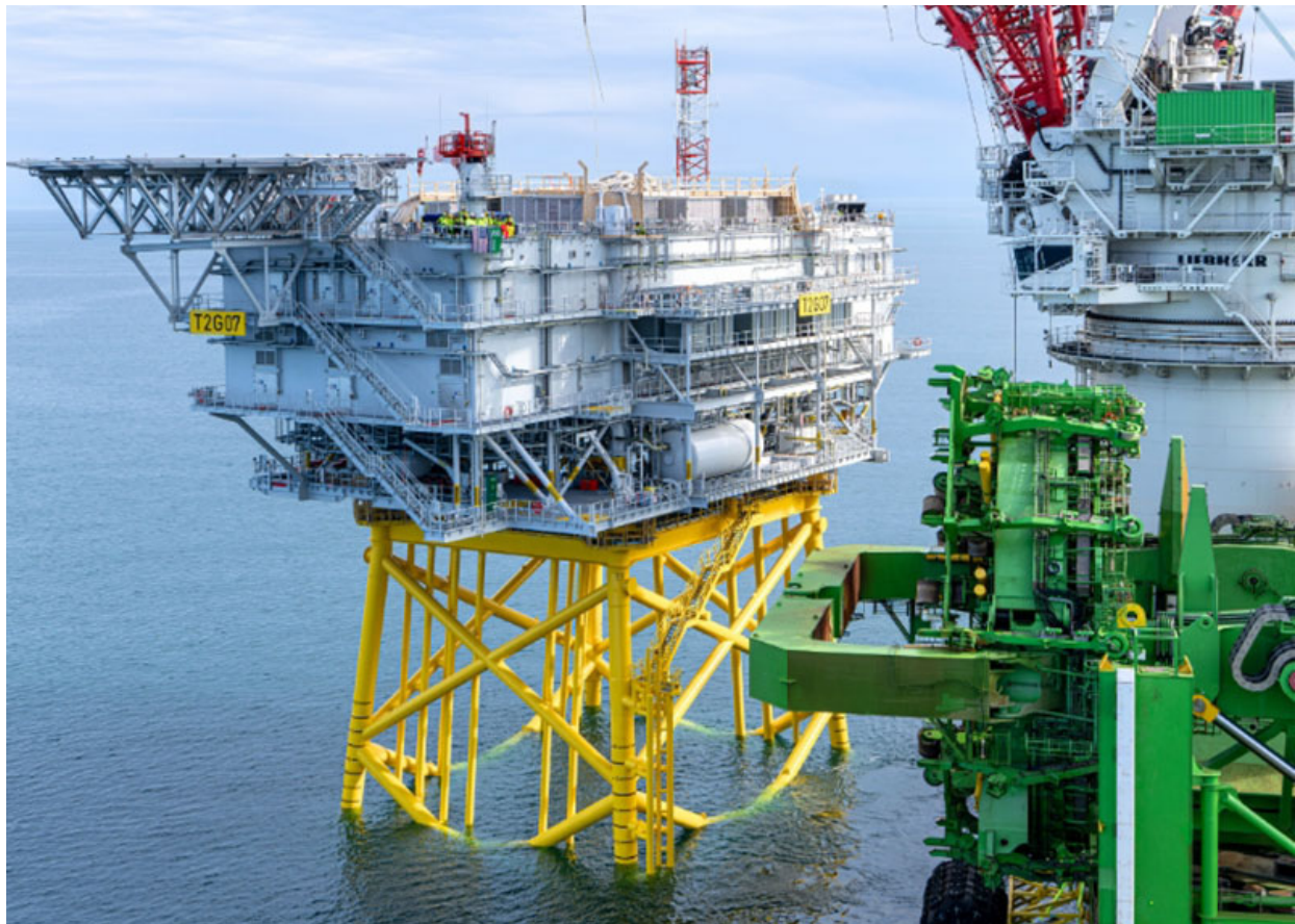
Figure 5: Completed OSS with topside
