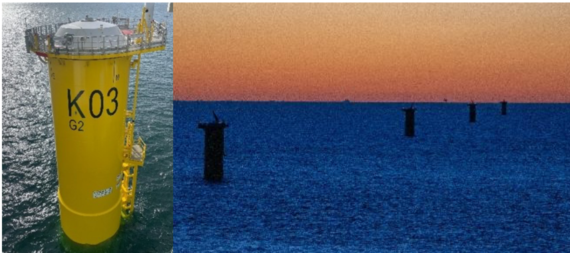
Figure 10: Temporary marine navigation lights on installed TPs
