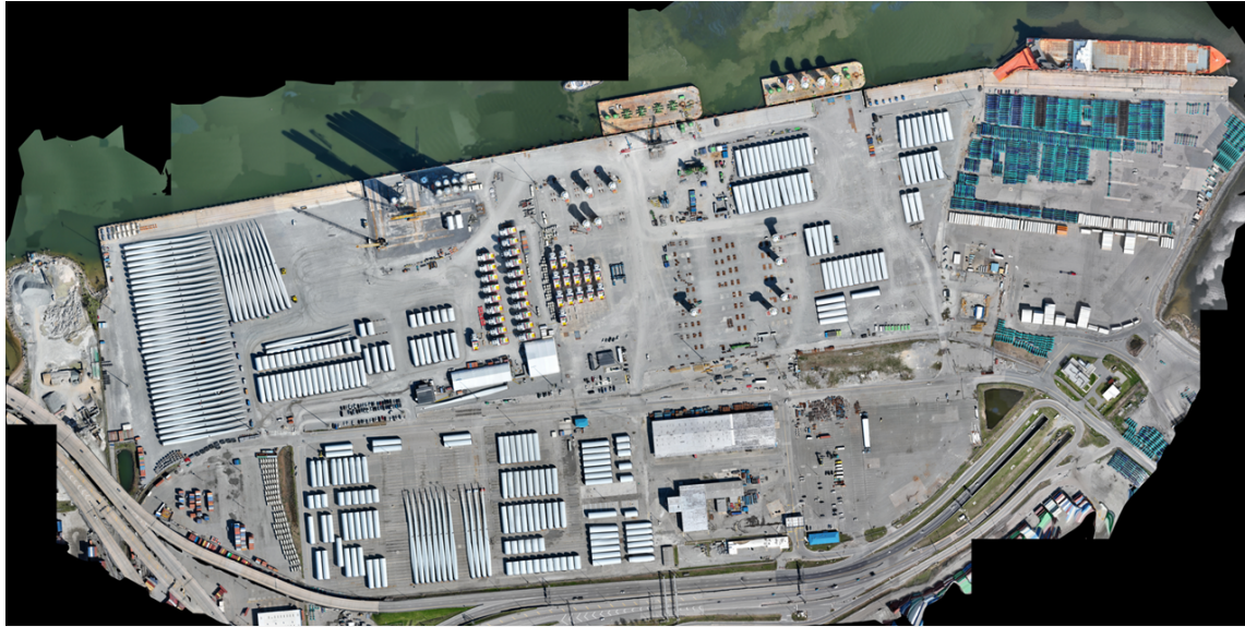
Figure 11: Portsmouth Marine Terminal – Staged WTG Components
