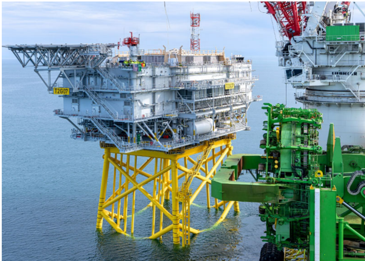
Figure 5: Completed OSS with topside
