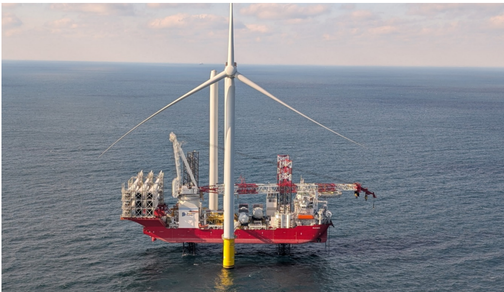
Image courtesy of Matthew Brooks First CVOW-C Wind Turbine Generator Installed By Vessel CHARYBDIS
