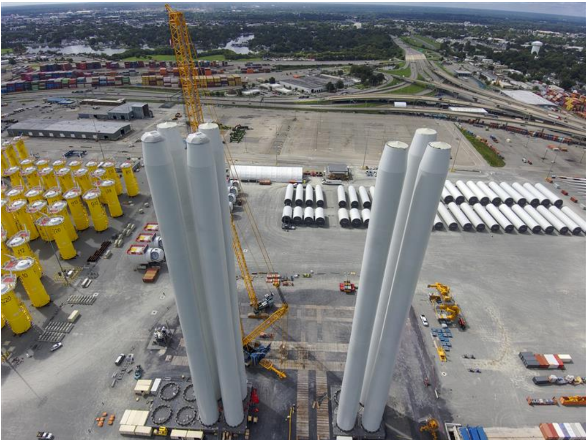
Figure 12: Completed Towers Quayside at Portsmouth Marine Terminal
