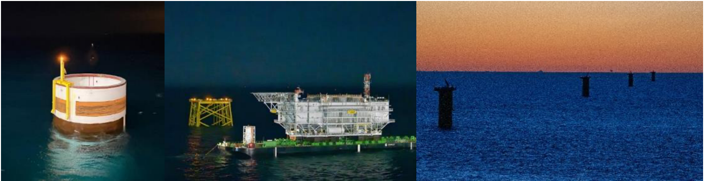
Figure 7: Lighted Navigation Lights on MP, OSS jacket foundations, and TPs
