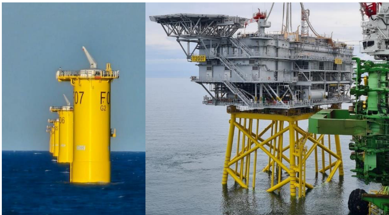
Figure 5: Installed TPs along “Row F” spaced 0.9-miles apart and Offshore Substation with Topside.
