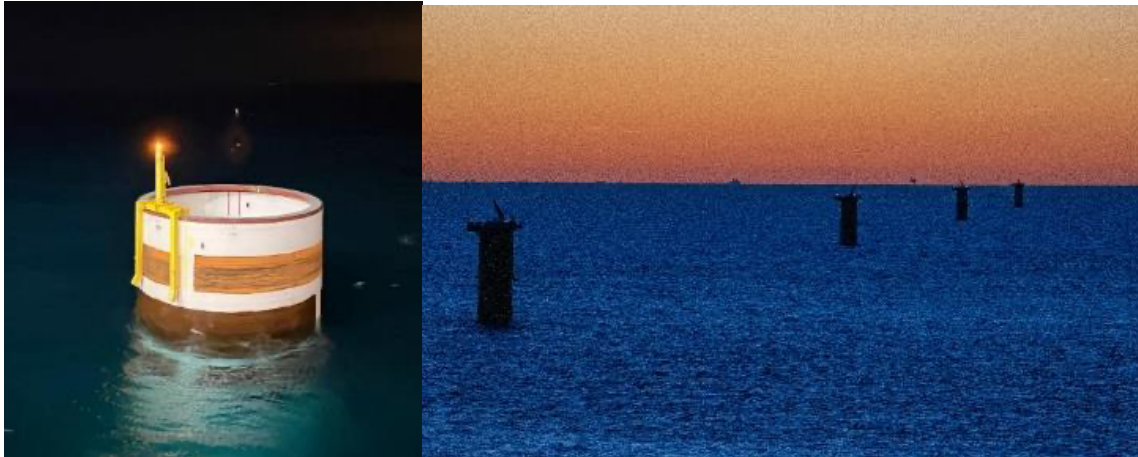
Figure 4: Lighted Navigation Lights on MP, OSS jacket foundations, and TPs
