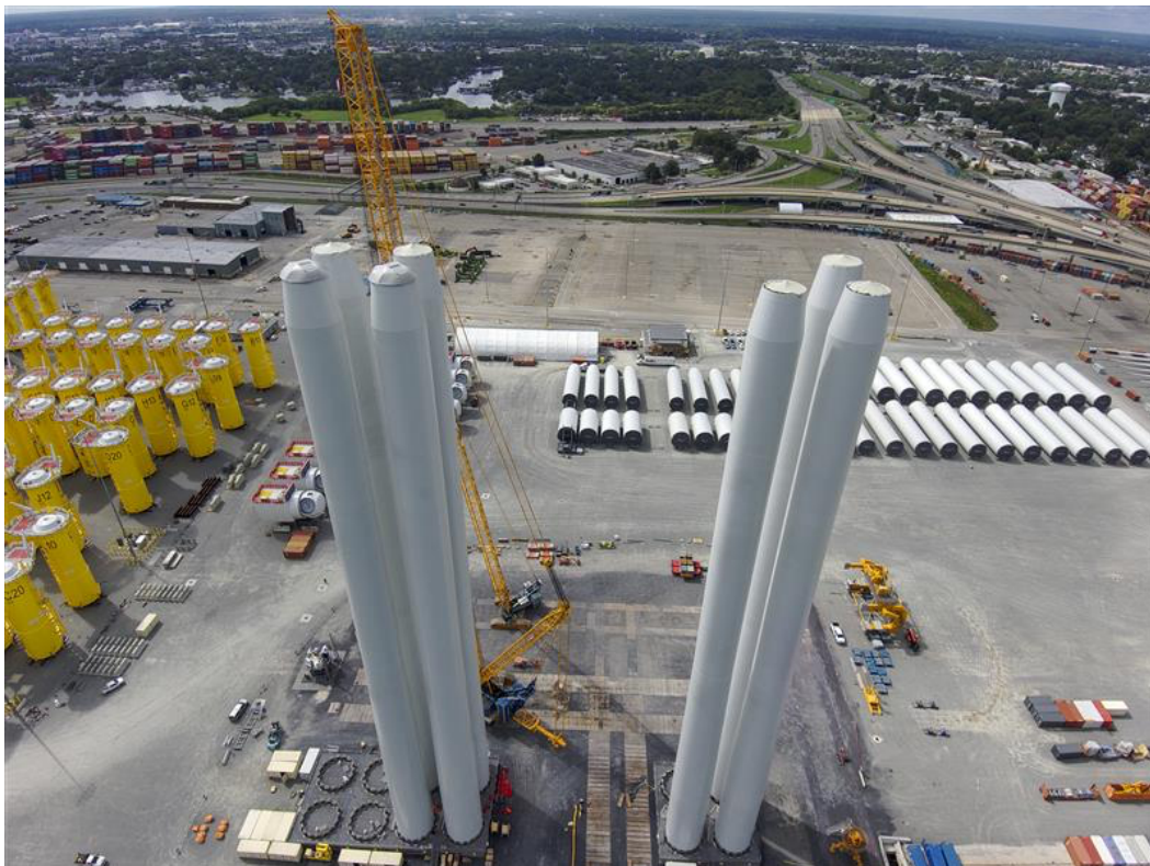
Figure 12: Completed Towers Quayside at Portsmouth Marine Terminal
