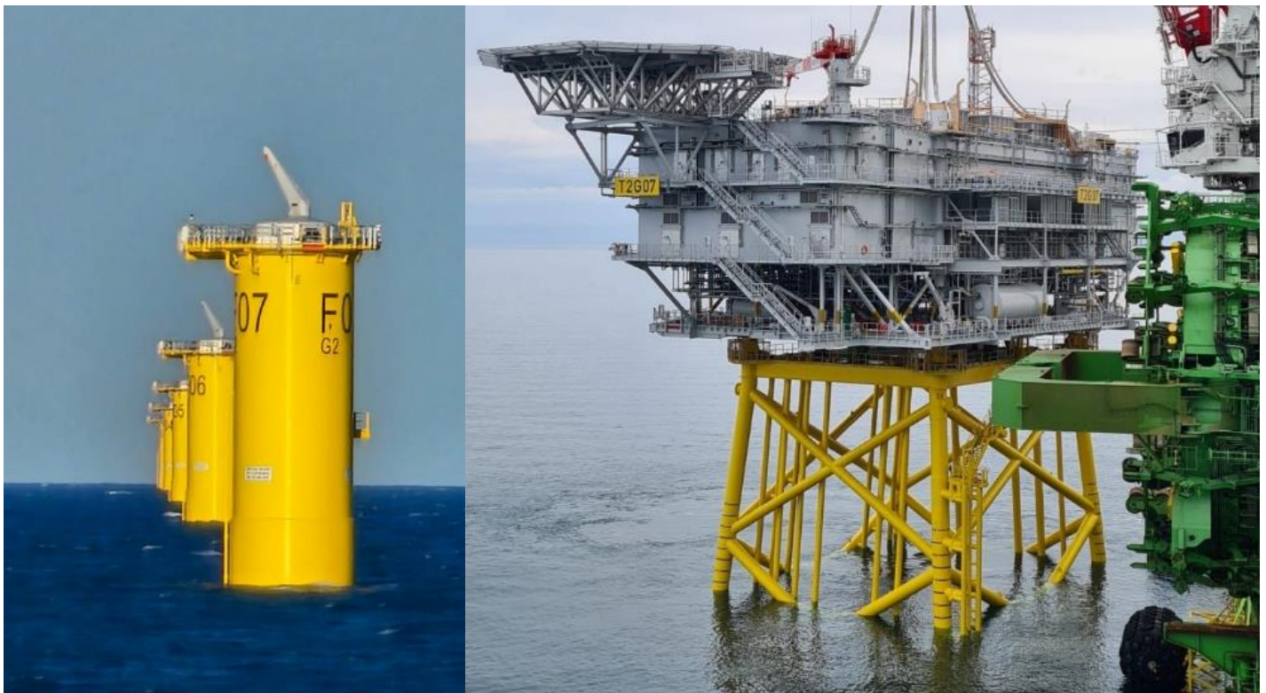
Figure 4: Installed TPs along “Row F” spaced 0.9-miles apart and Offshore Substation with Topside.
