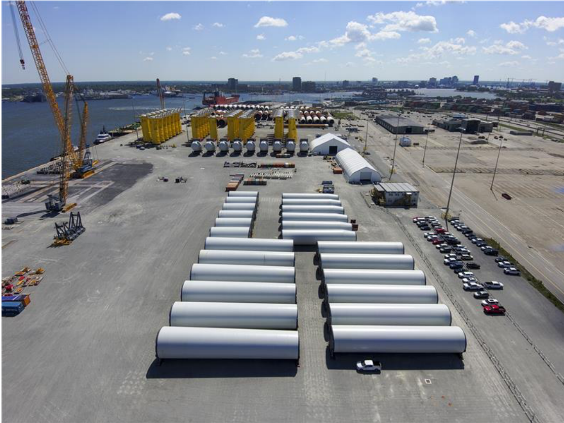
Figure 12: Portsmouth Marine Terminal – WTG Tower Sections Staged
